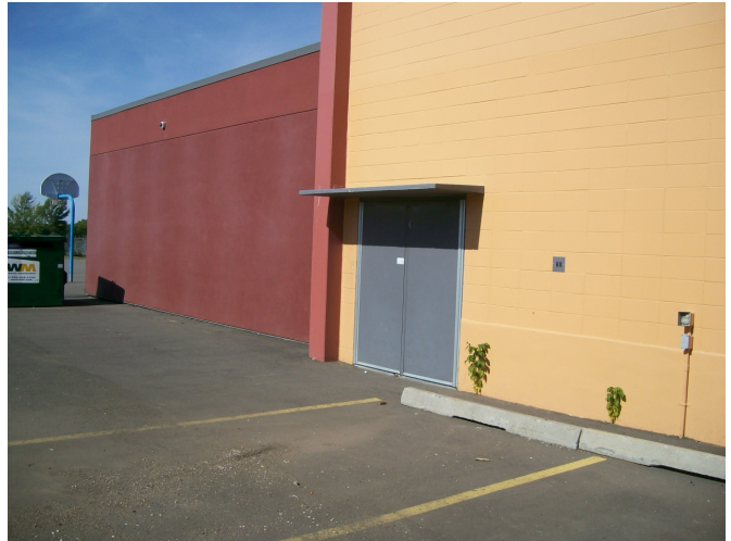
The precast concrete canopy for the gymnasium exterior door.:
