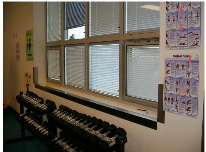
The exterior double glazed windows with integral blinds.
