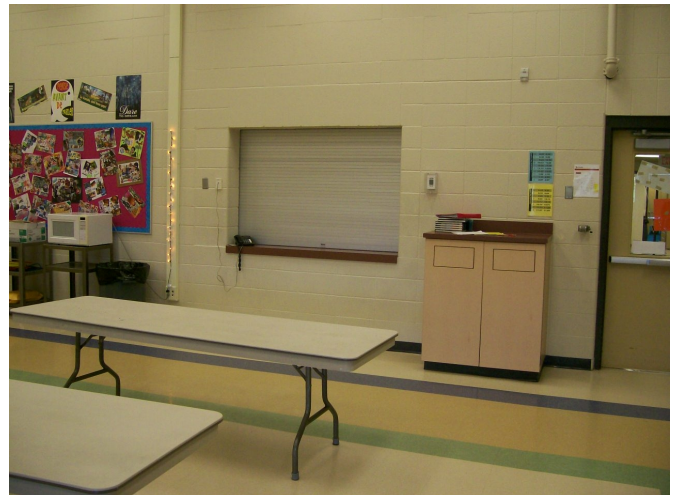
The metal overhead coiling door for the kitchen.
