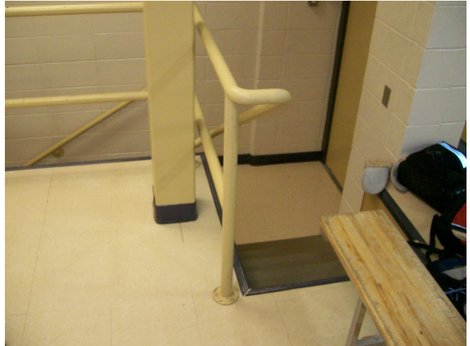
The steel pipe balustrades at the stage.
